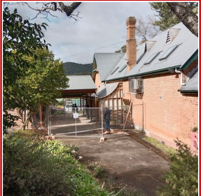
The long awaited building works are underway!
